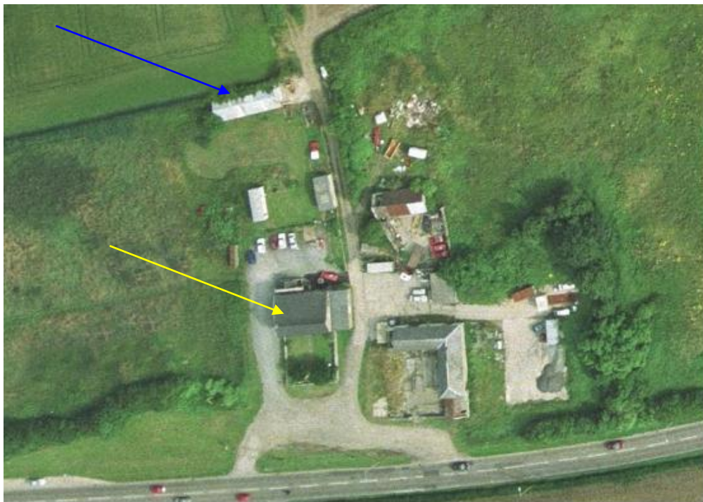
Figure 2 – detailed view of Welford Court Guesthouse. (Guesthouse arrowed yellow; outbuilding arrowed blue).
