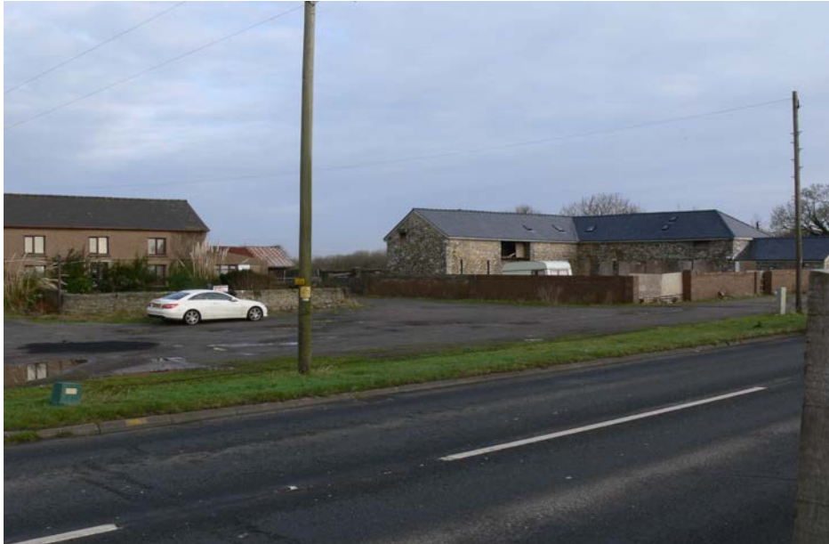
THE EASTERN BOUNDARY ACCESS LANE AND THE ADJOINING UNFINISHED RESIDENTIAL BARNS
