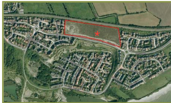
This aerial photograph shows the site north of Trem Echni with the surrounding Rhoose Point Development to date.
