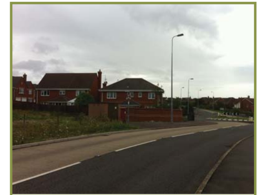
Below: Existing dwellings backing onto the site's eastern boundary, with the existing Gas Governor being served off Trem Echni.
