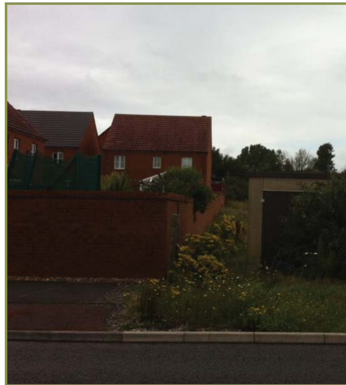
The site viewed from Trem Echni at the western boundary, showing existing dwellings predominantly backing onto the site.
