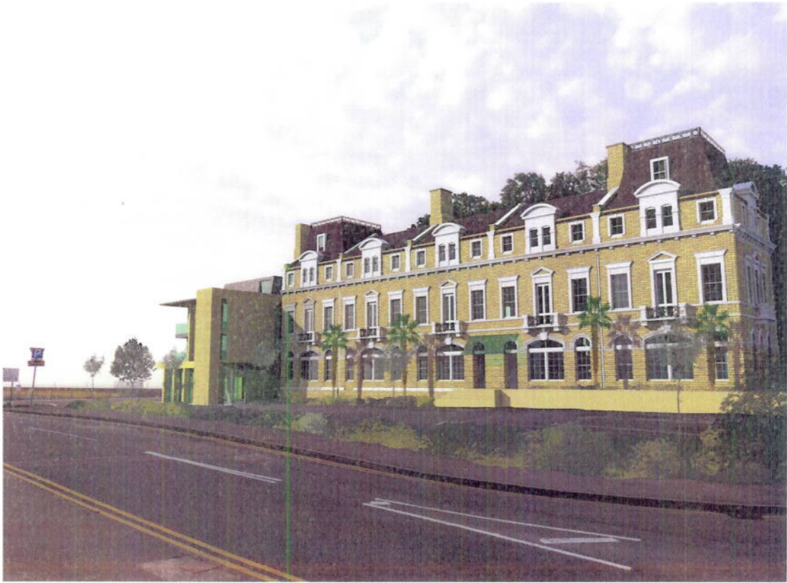
View of the Hotel from the roundabout
