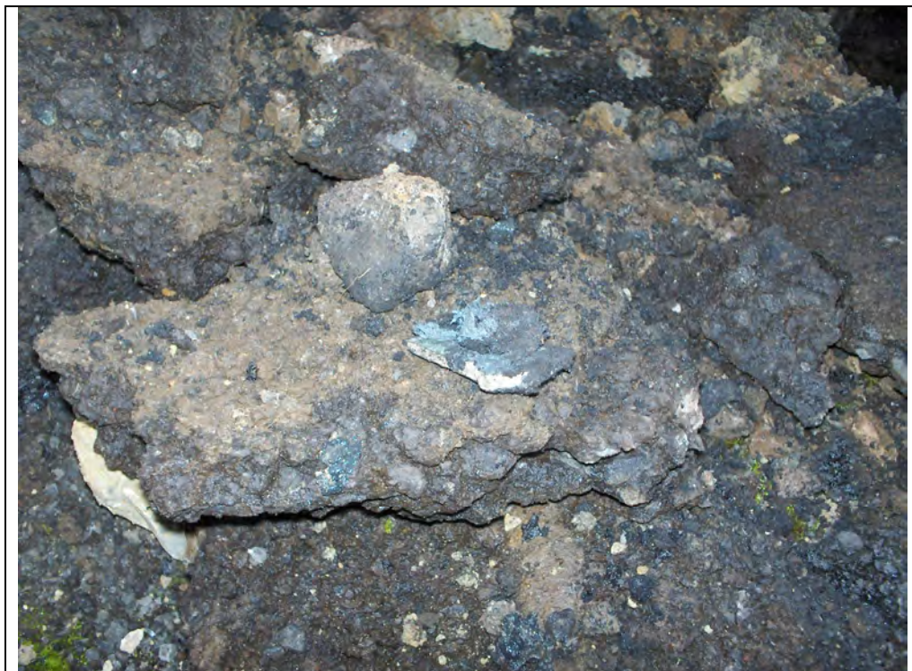
Plate 54: S/17633/04 Cement with Lagging applied (SQMTP37)
