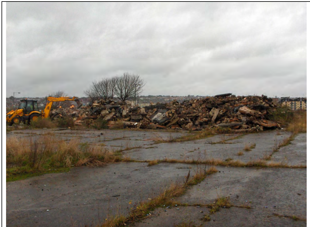
Plate 48: Stockpile A (oversize)
