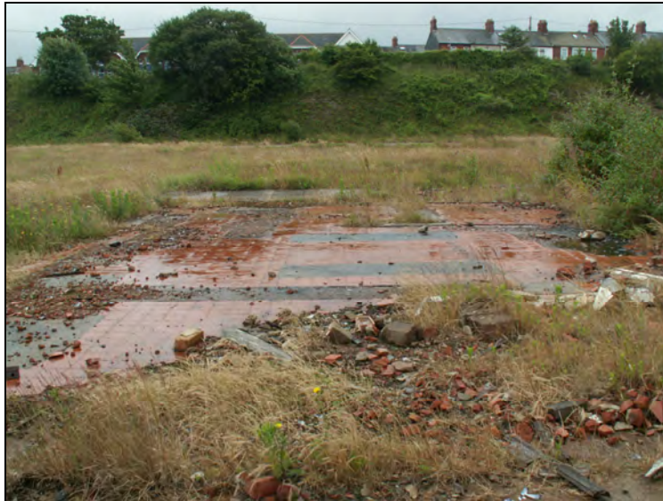
Plate G10: View to south of Floor slab of Oil Storage Terminal
