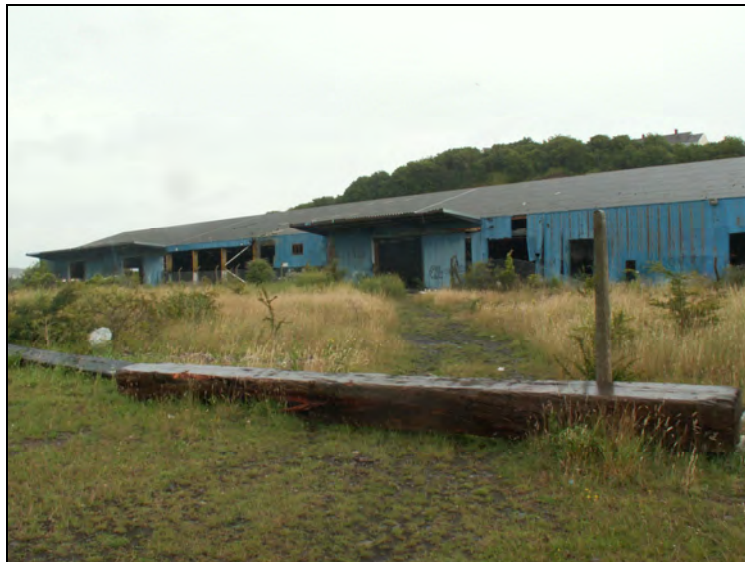
Plate G12: View to southeast of Warehouse
