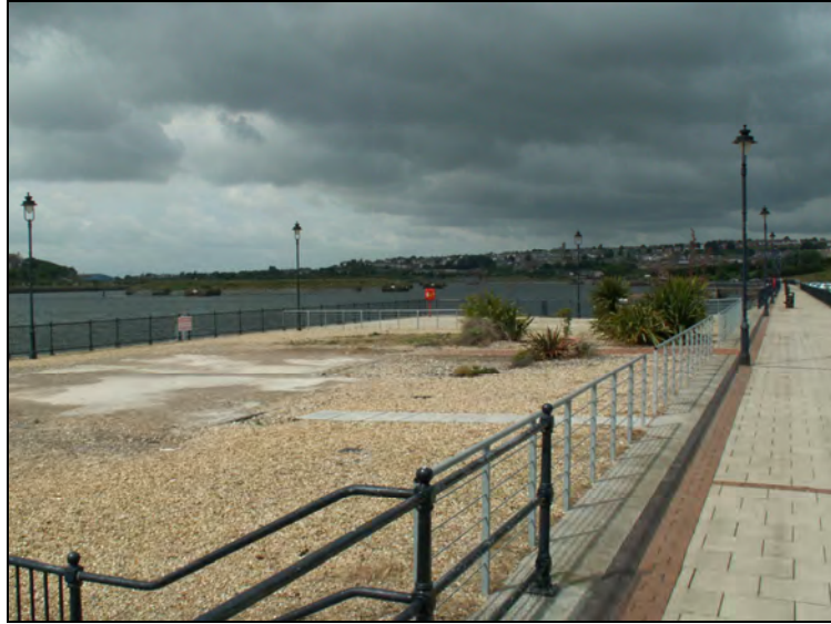
Plate G7: View to southwest of Castle Land Quay
