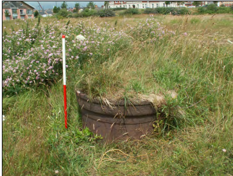
Plate G4: View to northwest of Metal pipe at East Quay
