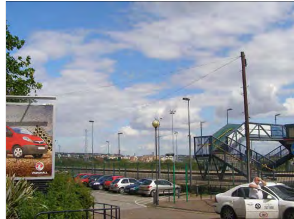
Barry Railway Station Facing East
