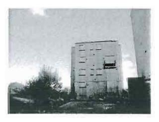
This is a single block, consisting of six, two storey flats with an internal staircase that serves all flats. They are of brick/block construction with pitched roofs clad with tiles.
