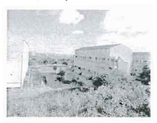
These are three identical blocks each with two with six, two storey flats. They are of brick/block construction with pitched roofs clad with tiles. There are concrete walkways leading to metal staircase at each end of the block. There is a large void space under the blocks.
