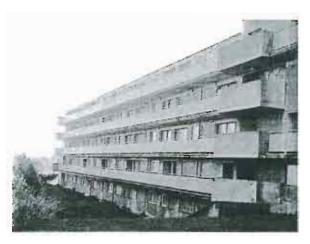
This block consists of 11 two-storey maisonettes on the ground floor landing and three landings of single storey flats above. There are also store cupboards located at ground level along the front of the block. There are stairways with associated service areas, constructed of brick and concrete. Internally the flats have brick/block external walls, with brick/block walls between flats. The partition walls and ceilings are of plasterboard and block construction.
