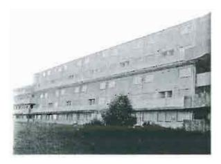
This block consists of 11 three-storey maisonettes on the ground floor landing and 11 two-storey maisonettes on the upper landing. There are stairways with associated service areas, constructed of brick and concrete. Internally the flats have brick/block external walls, with brick/block walls between flats. The partition walls and ceilings are of plasterboard and block construction.
