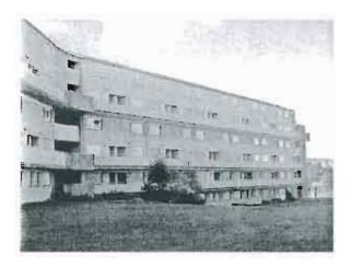
This block consists of 33 two-storey maisonettes on 3 landings. There are stairways with associated service areas, constructed of brick and concrete. Internally the flats have brick/block external walls, with brick/block walls between flats. The partition walls and ceilings are of plasterboard or block construction.
