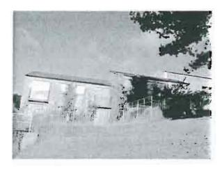
Four blocks, each containing, 8 single storey flats, with a hall and stairwell area shared between 4 four flats. They are of brick/block construction with pitched roofs clad with tiles. There are exterior storage areas of similar construction with flat felt covered roofs.
