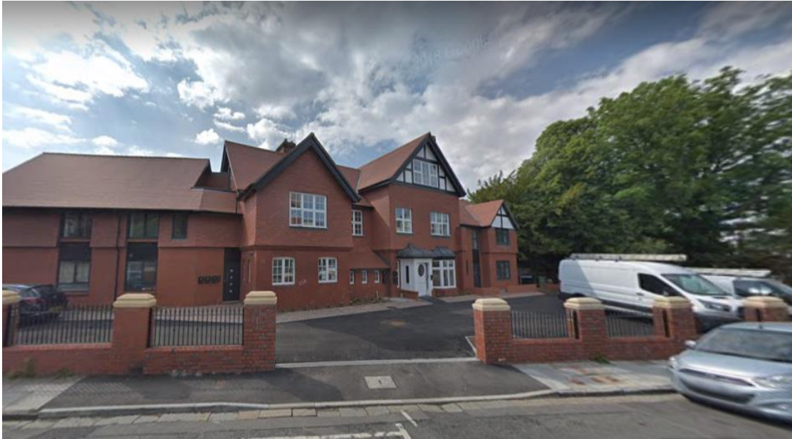
Street view from Rectory Road of site frontage
