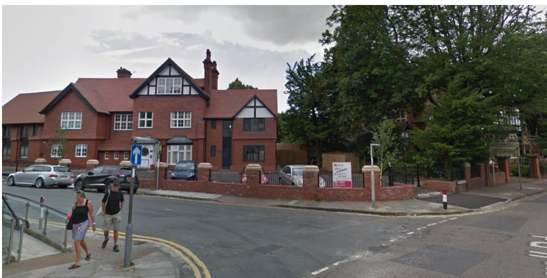
View looking south along Stanwell Road which highlights the previously modified nature of the area within which the structure would be sited when viewed from the north
