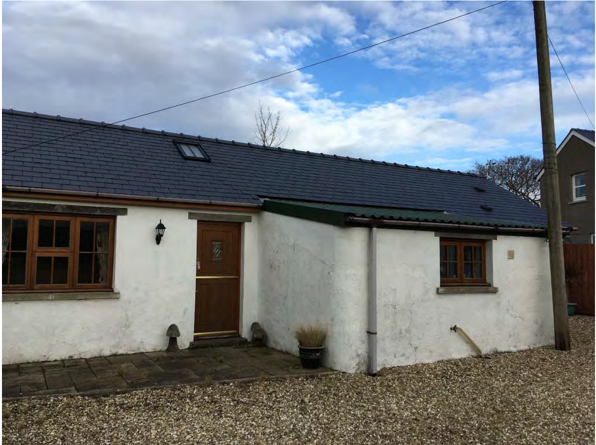
VIEW OF REAR ELEVATION OF APPLICATION SITE
