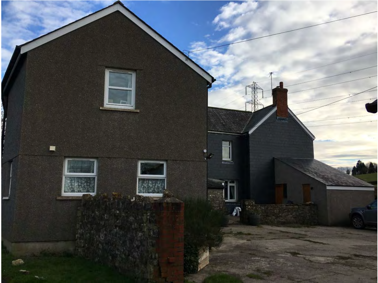
VIEW OF HEOL LAS FARMHOUSE – EXTENSIONS TO THE REAR VIEWED FROM ADOPTED HIGHWAY
