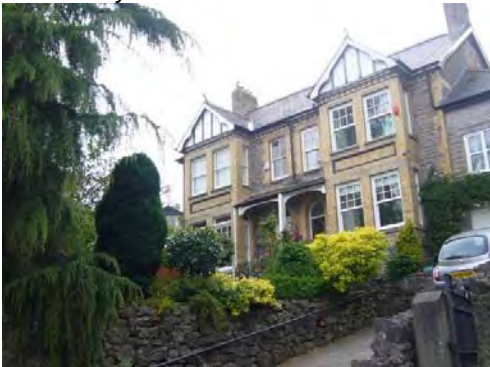
A pair of large semi-detached dwellings built soon after the arrival of the Barry railway.
