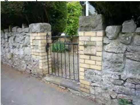
Stone wall and brick gate piers typical of the late 19 th century.
