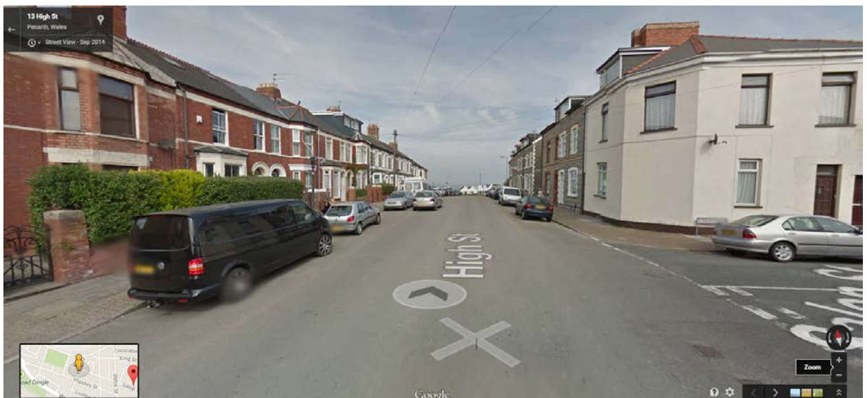
Examples of large flat roof dormers on the front roof slope on High Street adjacent to the appeal property.
