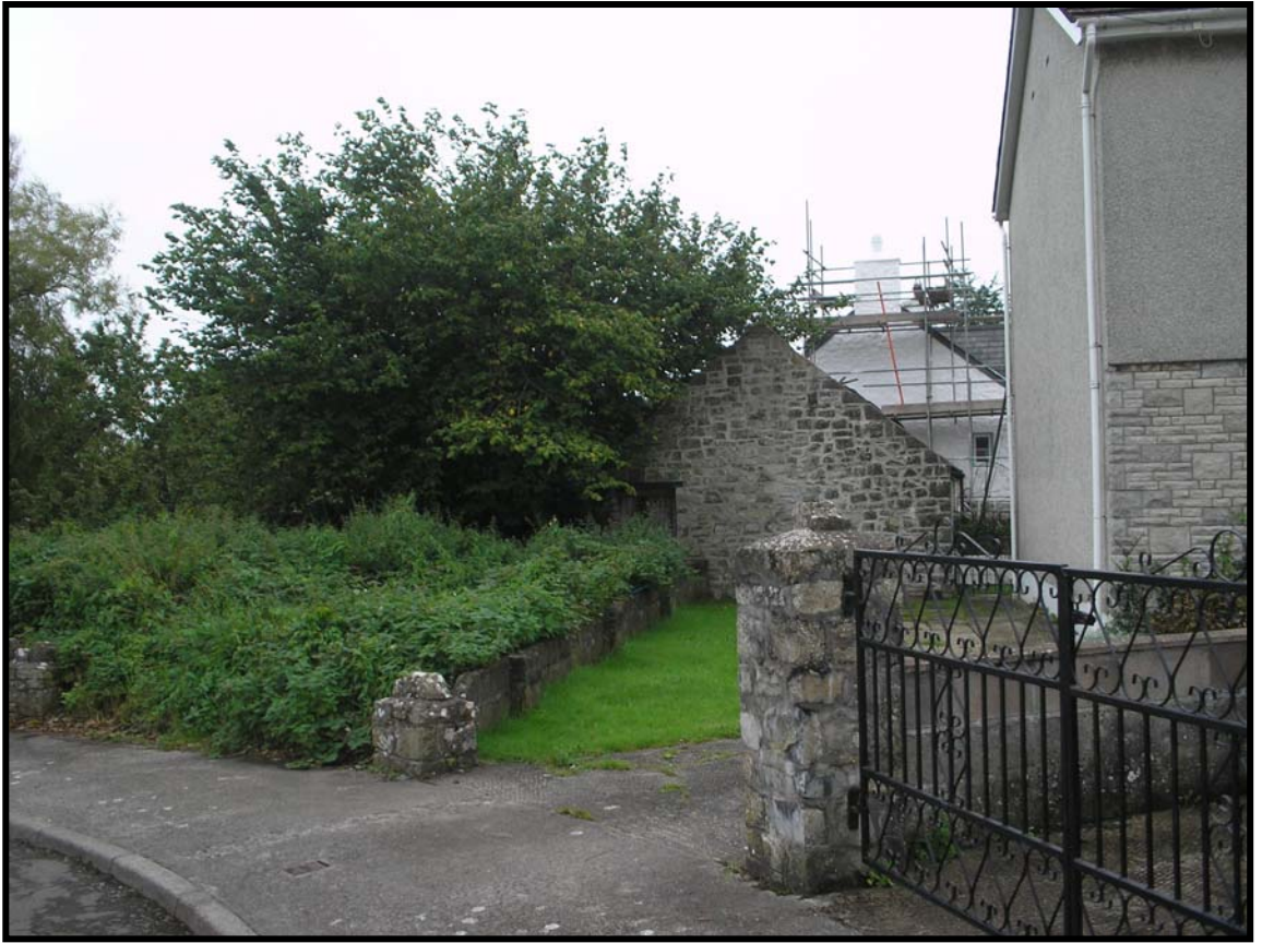
Photo No. 1: Appeal site showing proximity to gable end of Grade II listed Swimbridge Farmhouse
