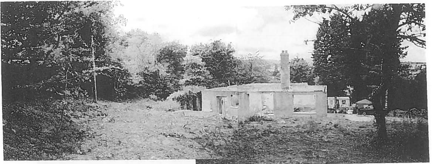
⑤ VIEW OF SITE LOOKING NORTH
