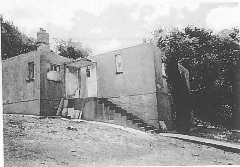
⑩ EXISTING REMAINS OF BURNT OUT HOUSE TO BE DEMOLISHED.
