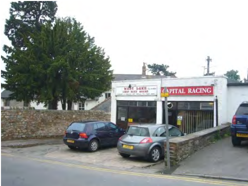
Flat-roofed single storey shops are out of keeping with the historic character of the conservation area.
