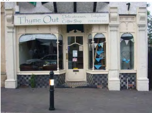
A well preserved and finely detailed early 20 th century shopfront at no. 5 Elm Grove Road.
