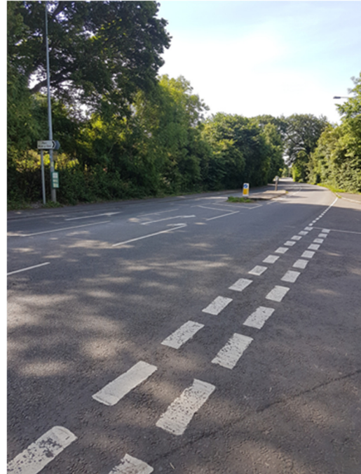
Photograph 5: A4055/ Cardiff Road looking south from Northbound Bus Stop
