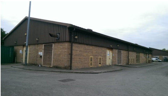
Figure 12: Example of building
