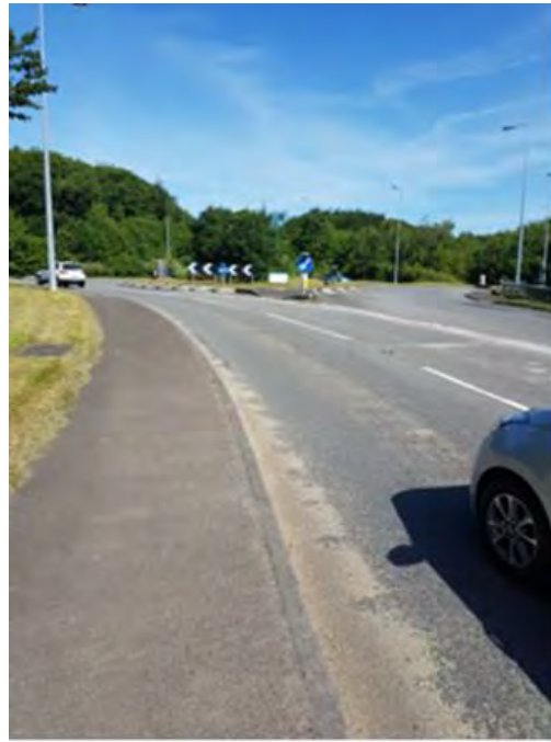
Photograph 3: A4050 Port Road Roundabout
