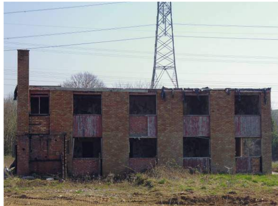
Plate 18: Building 5 – Western elevation
