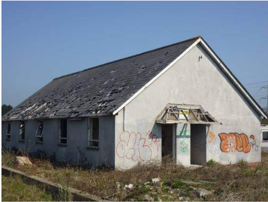
Plate 1: Building 1 – South-east elevation
