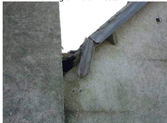
Plate 24: Hole in the bargeboard of the western elevation of building 6, near the bell tower
