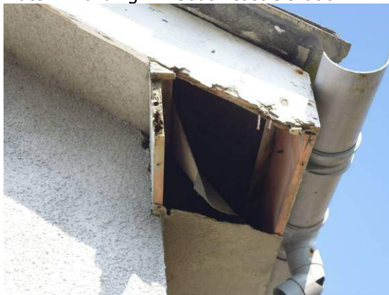
Plate 3: Access into soffit box of building 1
