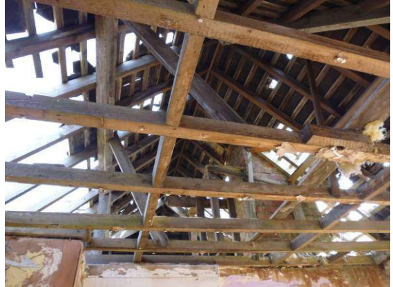
Plate 8: Internal roof structure of building 2
