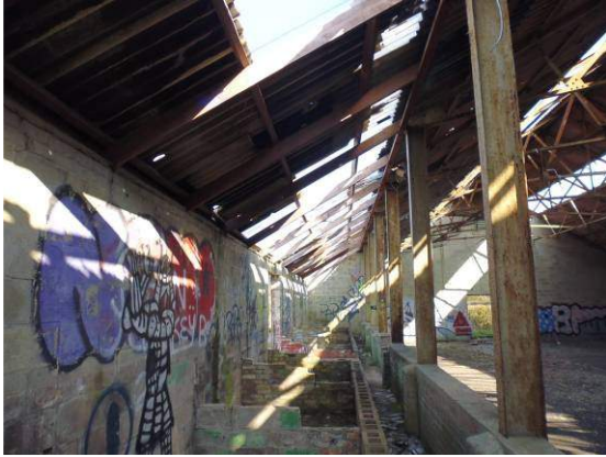
Plate 35: Internal view of building 7 showing high number of large holes in roof
