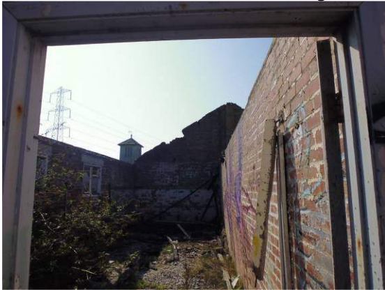
Plate 15: Internal view of central portion of building 4
