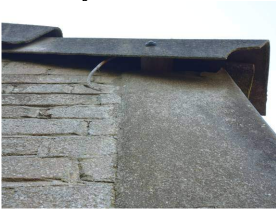
Plate 37: Gaps beneath asbestos bargeboards at northern elevation of building 7
