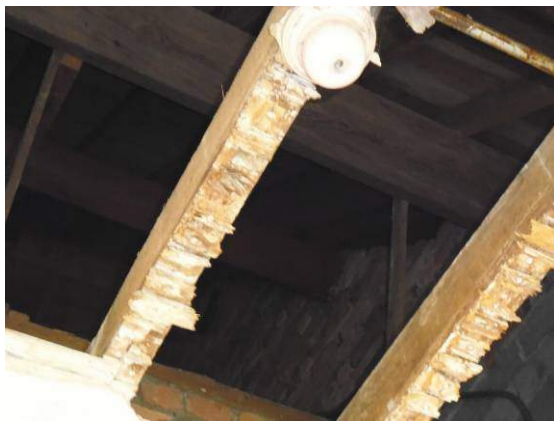
Plate 29: Internal view of void
