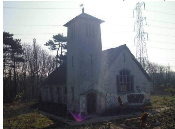
Plate 22: Building 6: North-western elevation
