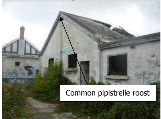
Plate 16: Building 4 – Roost Access (2012)
