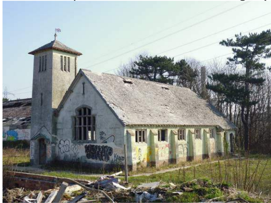
Plate 21: Building 6: South-western elevation
