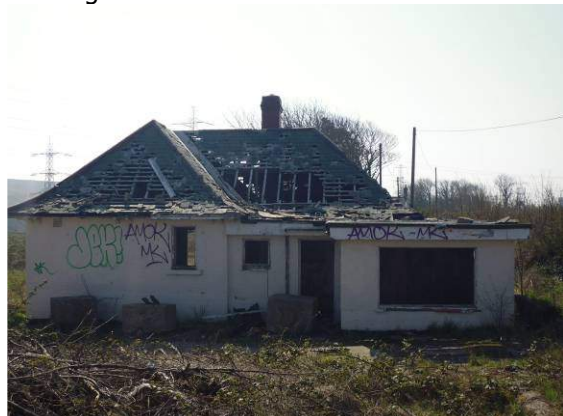
Plate 6: Building 2 - Northern elevation
