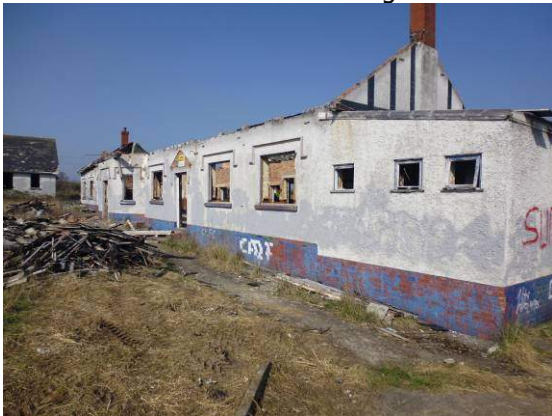
Plate 9: Building 3: South-east elevation
