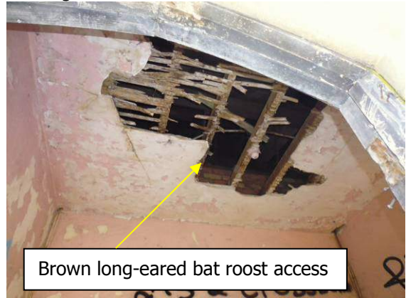
Plate 28: Access to roof void at east of building 6 (2012)
