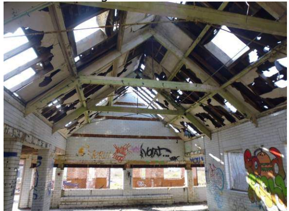
Plate 12: Internal view of roofspace of northern section of building 3
