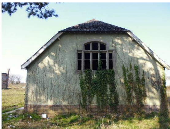
Plate 25: Building 6: Eastern elevation
