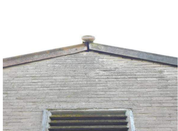
Plate 38: Moderate sized gap at apex of northern elevation wall
