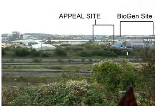
Photograph 5, View of site from Dock View Road/ Castleland Street Junction
