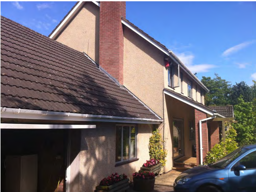
Photograph showing front elevation
