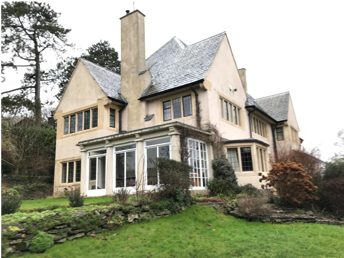
3 Current Photo of Lon Twyn with timber framed doors & windows enclosing loggia
